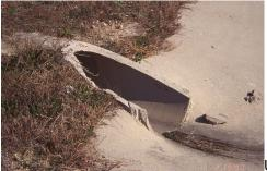
Use **Beveling of Pipe End** (719-610-00) when specified in the plans or special provisions. Beveled ends may only be used on flexible pipe up to 24" diameter and on rigid pipe up to 60" diameter. When beveling of pipe ends is specified on flexible pipe larger than 24" diameter, install pipe straight headwall, pipe end structure, flared end section, or wingwall section. Use factory fabricated beveled ends for all pipe types unless approved by the Engineer.
