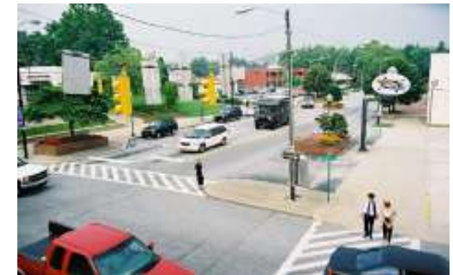
Small curb return radii and curb bulb-outs at intersections shorten the time and distance that pedestrians are exposed to traffic in intersection and mid-block
