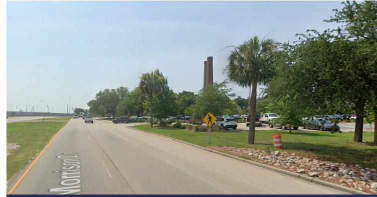
Missing sidewalks on Morrison Drive
