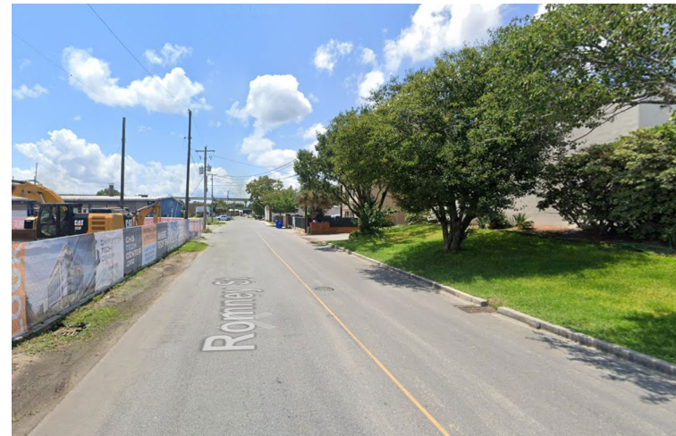
Missing sidewalks on Romney Street
