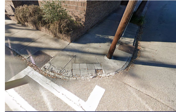
Sidewalk ramp at East Bay St and Wentworth Ave
