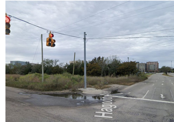
Missing sidewalk, crosswalks, and flooding issues on Hagood Avenue
