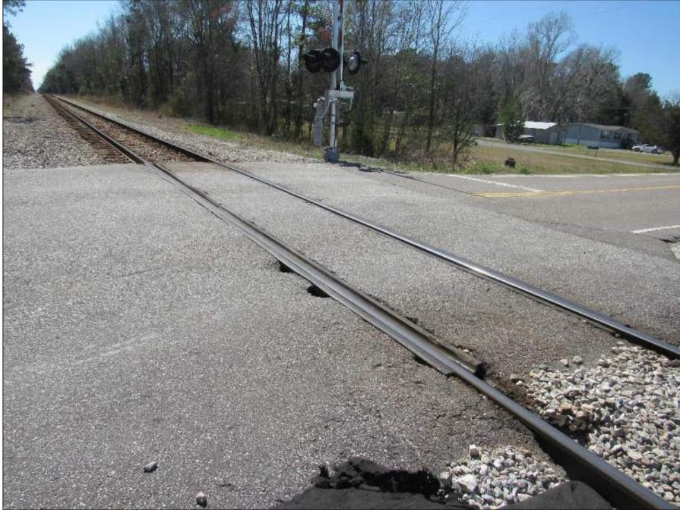
**Figure 6 – Gaillard Road Rubber Crossing Surface (Low Clearance Scraps and Pavement Spalls)**
