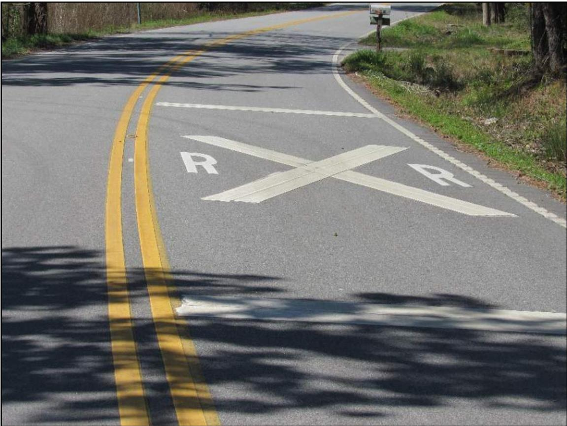
**Figure 7 – Oakley Road West Approach Railroad Crossing Pavement Marking**
