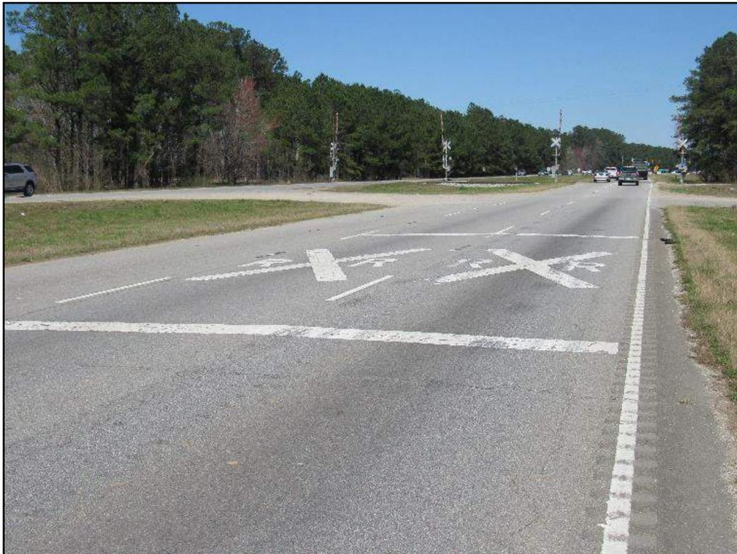
Figure 12 – US-52 Northbound Roadway Pavement Markings Looking North
