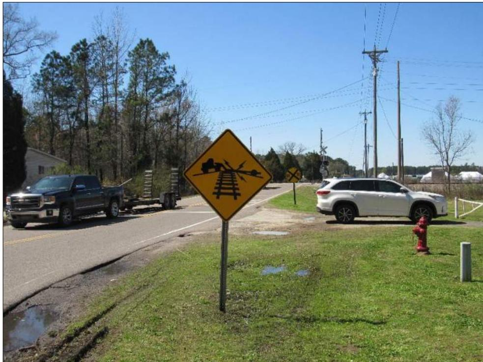
**Figure 7 – Gaillard Road East Approach Advance Warning Signs**
