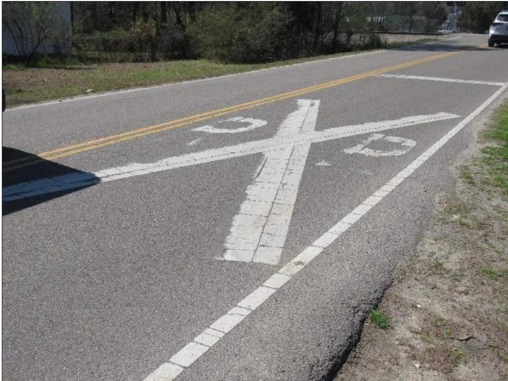
**Figure 9 – Gaillard Road East Approach Railroad Crossing Pavement Marking**
