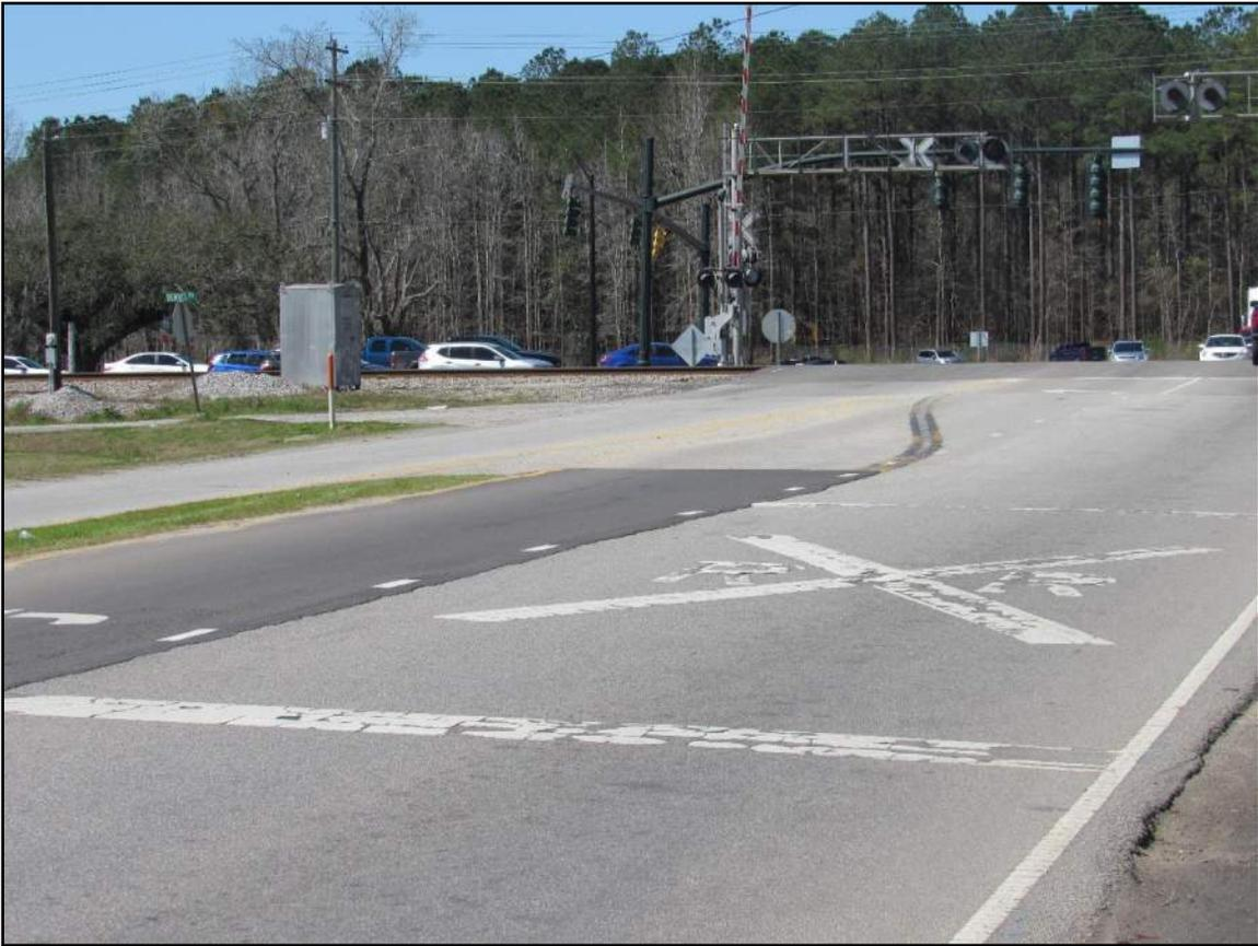
Figure 12 – Montague Plantation Boulevard East Approach Railroad Crossing Pavement Marking Looking West
