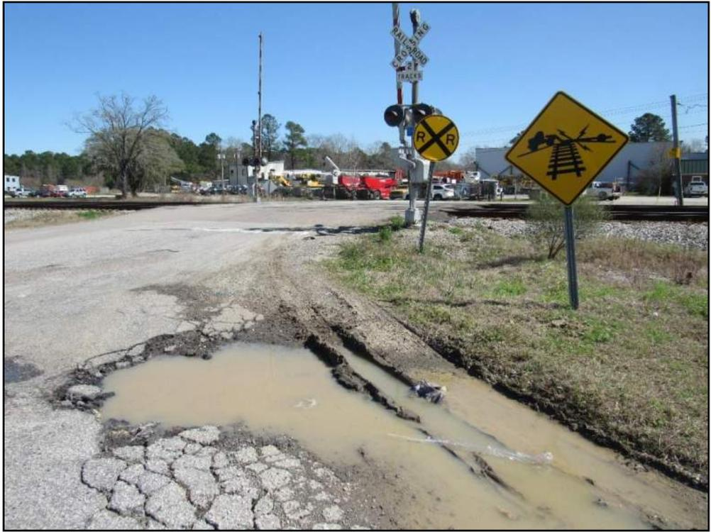
Figure 5 – Medway Road West Approach Pavement Spalls and Advance Warning
