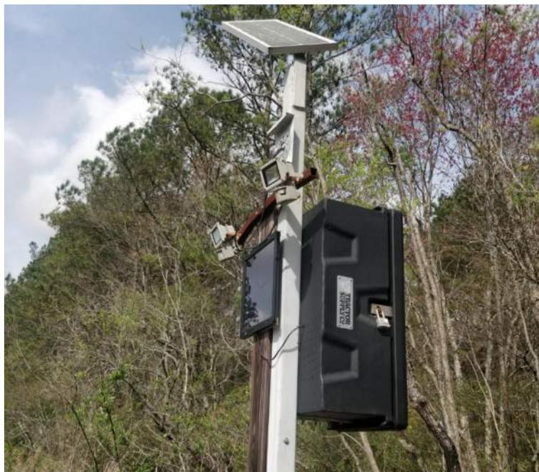
**Figure 4 – Mount Holly Plantation Lane – Train Facing Interconnected Signal Close Up**
