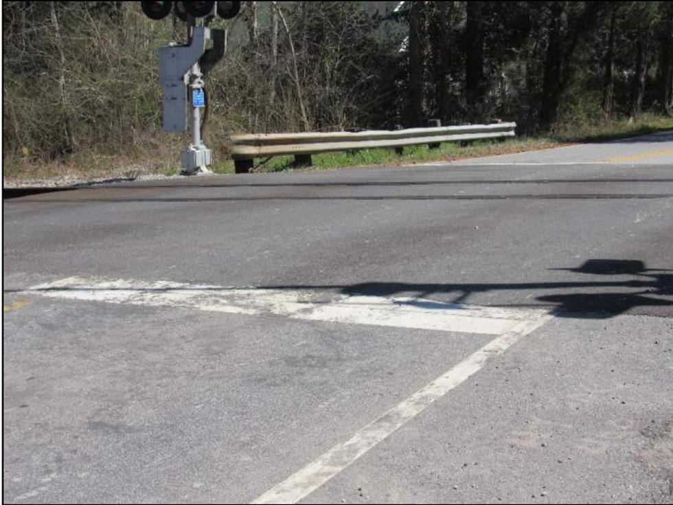
**Figure 8 – Oakley Road East Approach Stop Bar Pavement Marking**
