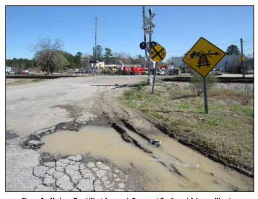
Figure 5 – Medway Road West Approach Pavement Spalls and Advance Warning
