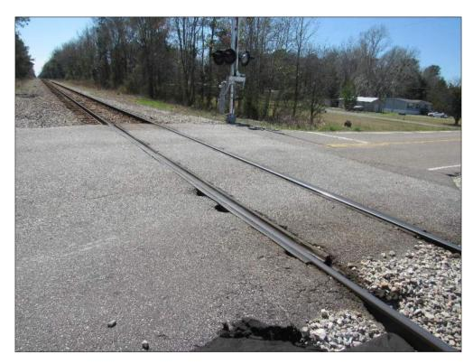
Figure 6 – Gaillard Road Rubber Crossing Surface (Low Clearance Scraps and Pavement Spalls)
