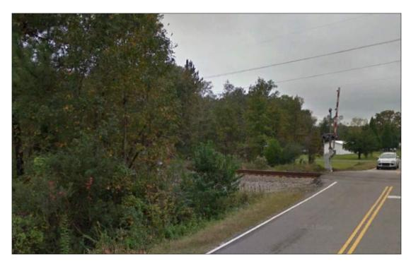
Figure 12 – Gaillard Road Southeast Quadrant Sightline Obstructed
