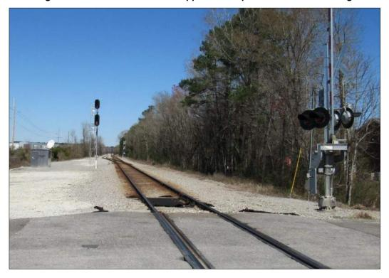
Figure 11 – Gaillard Road North Approach – Ballast Fouling Track Surface
