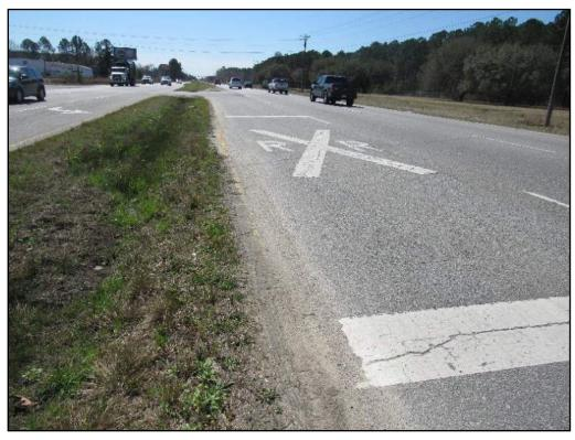
Figure 7 – US 52 North Approach Railroad Crossing Pavement Marking Looking South Approach
