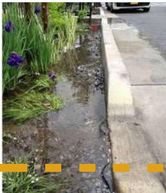
*right.* Bioretention within the right-of-way
