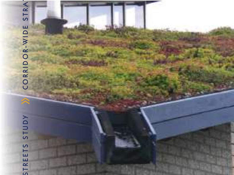
**Green roofs** are covered with vegetation and a growing medium installed over a waterproof membrane. Green roofs absorb rainwater, provide insulation, create wildlife habitat, and help to mitigate urban heat island effects and lower urban air temperatures. Green roofs become more financially viable within higher intensity and space-constrained town center areas, and should be considered as a demonstration project for new municipal buildings.
