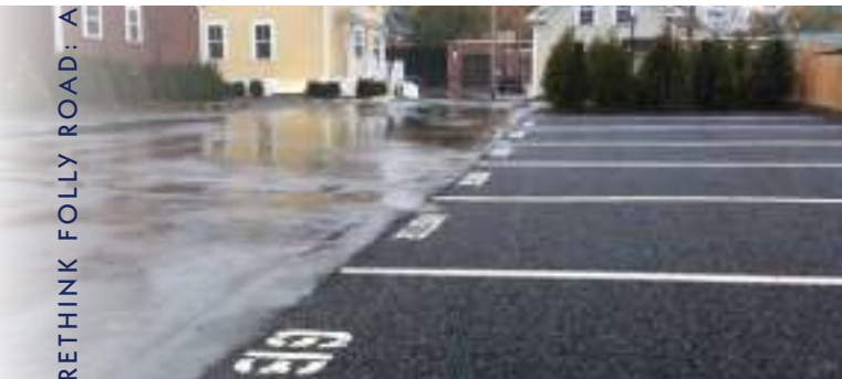
top: Tree box filters – Source: Stormtree middle: Green Roof – Source: Wikimedia Commons bottom: Permeable pavement - private parking and public right-of-way applications
