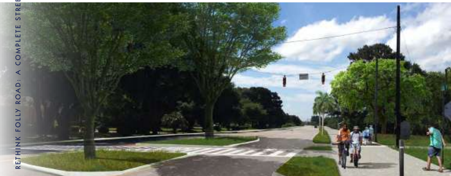
below: Proposed reconfiguration of Folly Road to three lanes; without the outside travel lane, landscaping and a shared-use path can be installed.
