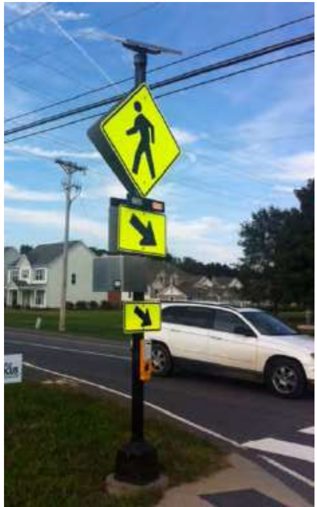
Rectangular Rapid Flashing Beacons (RRFB) utilize a warning yellow LED stutter flash light bar within the standard crossing sign assembly. They have proven an increased motorists yield rate versus other flashing beacon warning systems. They are especially useful at multilane crosswalks.
