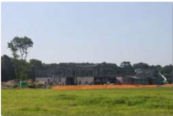
Construction of First Baptist Athletic Complex (Source: BCDCOG Staff)
