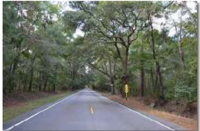
Trees close to Bohicket Road have reflective signs and devices to improve safety (Source: SCDOT)
