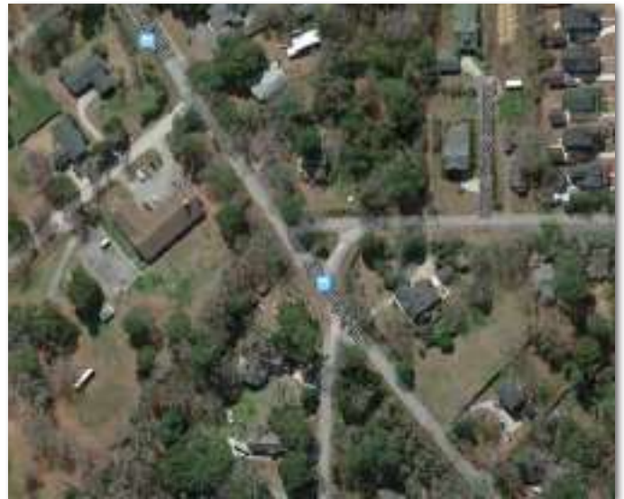
Riverland Drive at Woodland Shores Road Intersection. (Retrieved on May 28, 2014 from www.google.com/maps )
